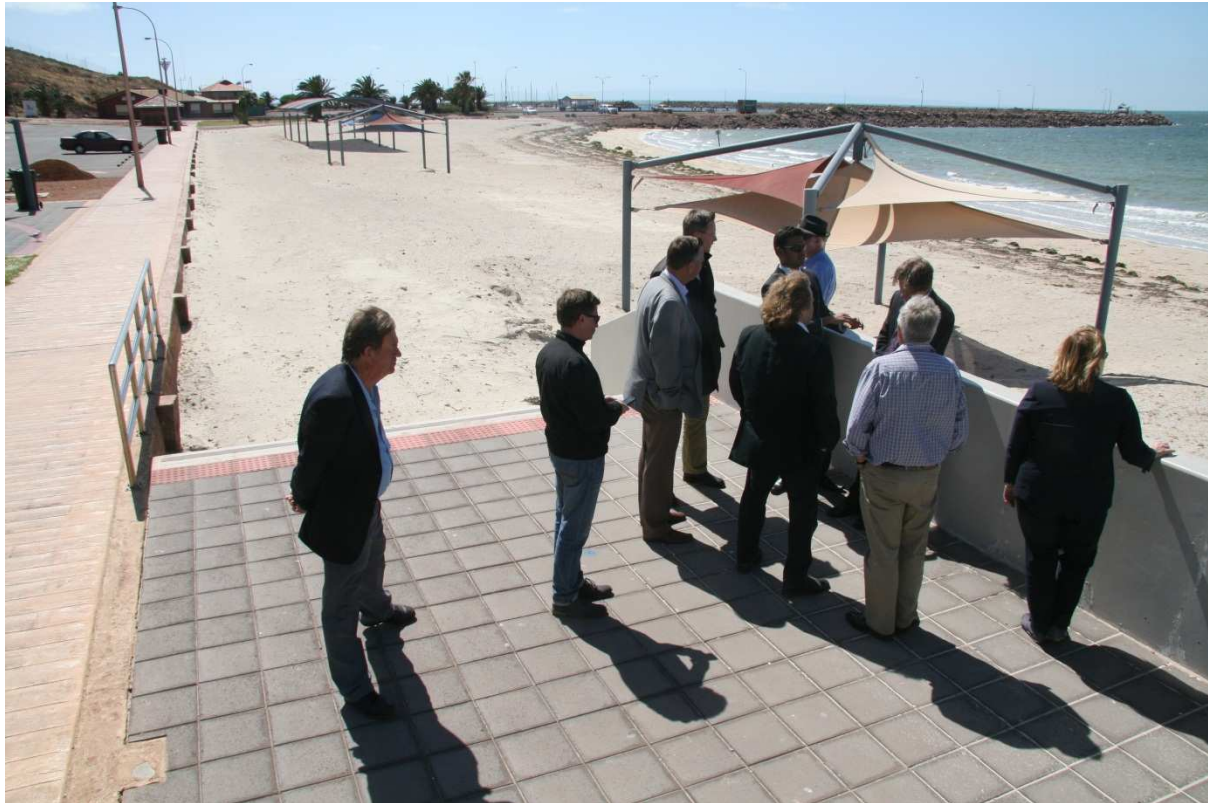
Figure 33: The reconstructed sea wall which was damaged by a king tide
