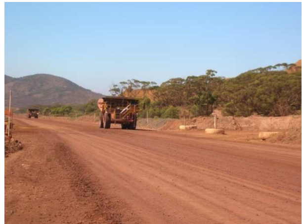
Figure 6: 'before' and 'after' photographs of roads treated with magnesium chloride to reduce fugitive dust from roads (Arrium 2013, p7)
